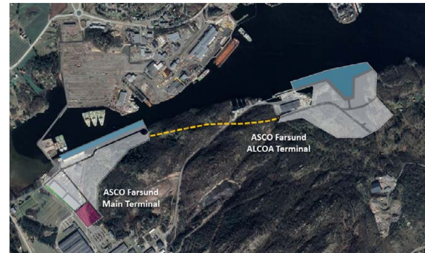
Potential Future Expansion at ASCO's location in Farsund, Norway.
