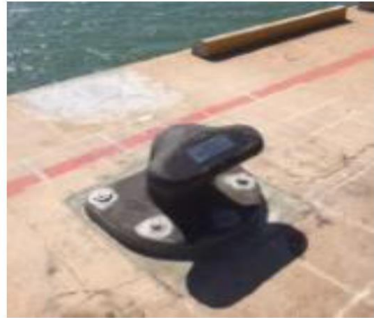
Derated Bollard, Single Mooring Line Berth 3
