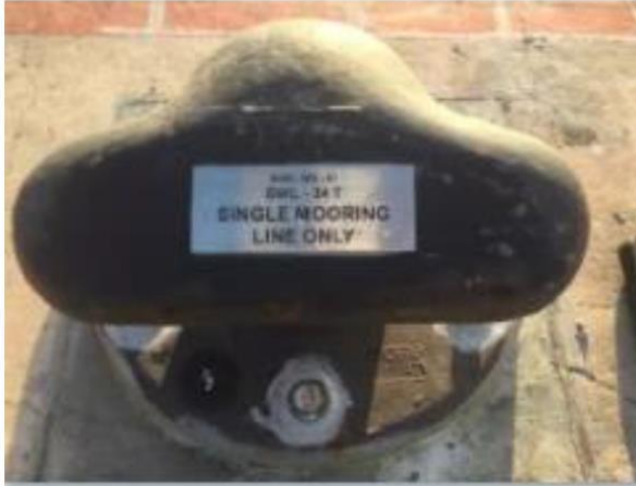
Derated Bollard, Single Mooring Line Berth 3
