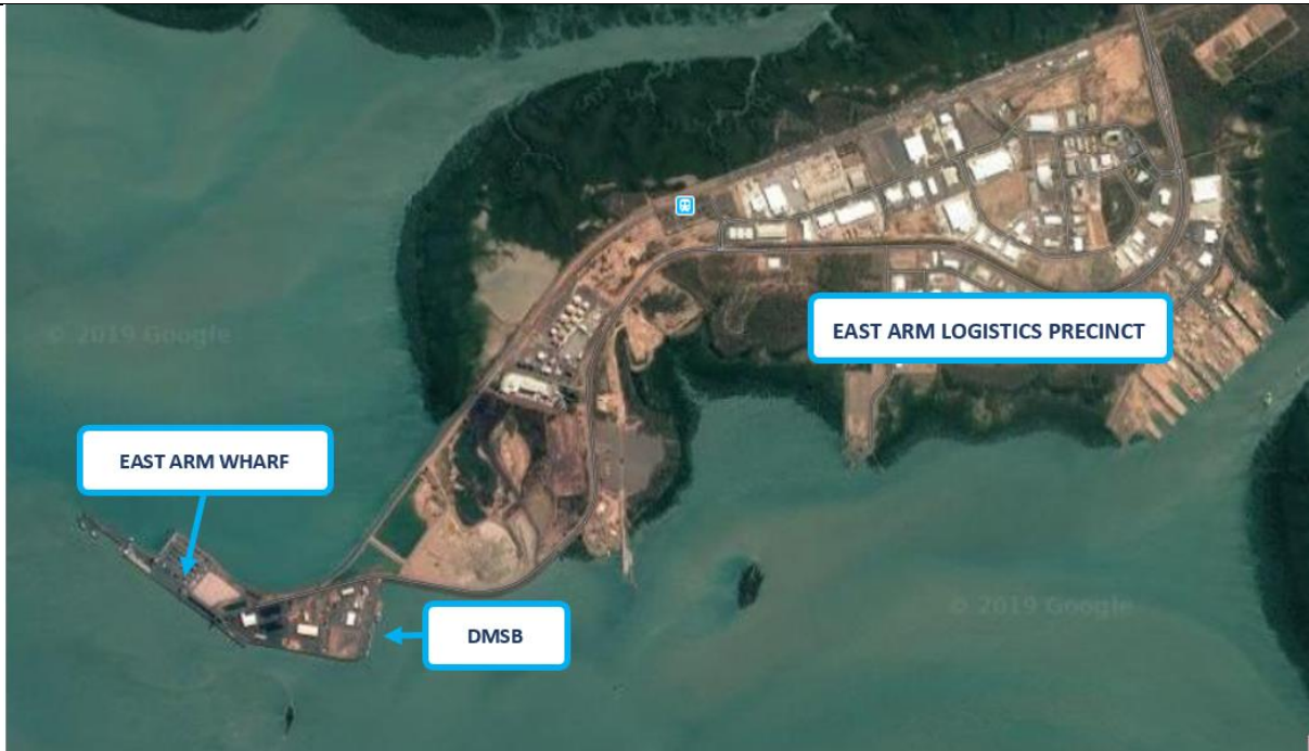
Figure 2 - DMSB is located alongside East Arm Wharf, approximately 2.km from East Arm Logistics Precinct.
